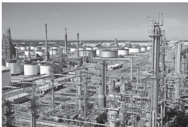
FIGURE 21.2 Process piping transports fluids between storage tanks and processing equipment at this oil refinery.
