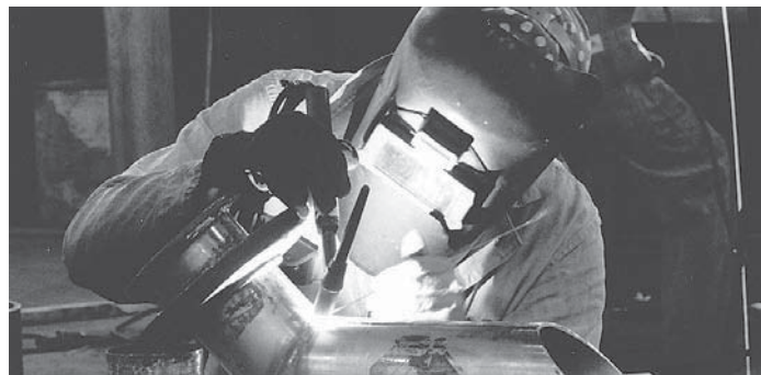
FIGURE 21.60 Pipe fitter welding a piping spool assembly. Courtesy Alaskan Copper Works
